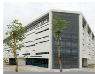
R&D Center in Fujitsu General Engineering (Thailand)
